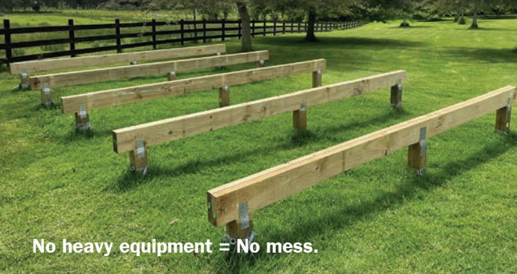
Easier to line up piles.
